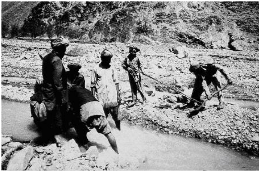
Photo 3. Reconstructing a traditional diversion weir
