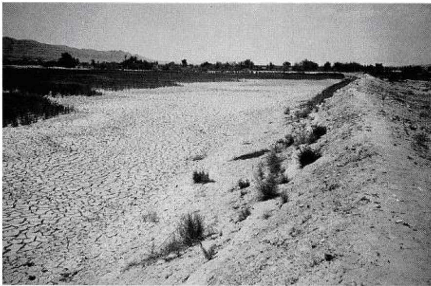
Photo 1. Earthen bund for water harvesting
